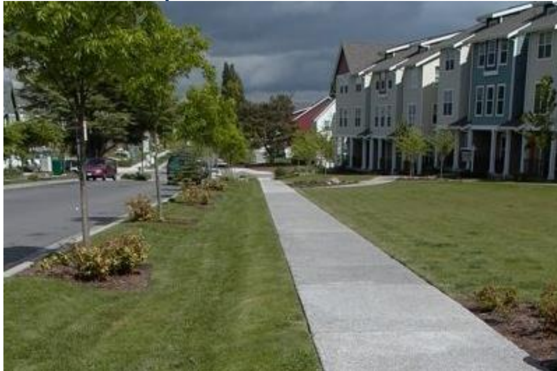
Example Permeable Concrete Sidewalk
