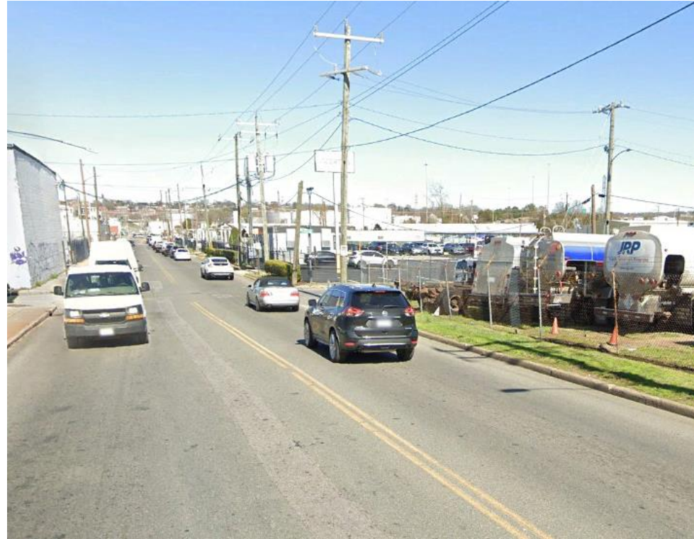
Photo looking east from 700 block of Maury Street adjacent to Hopper Lofts
