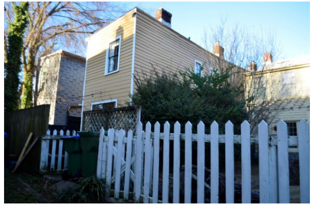
Figure 6. View of the rear, two-story addition at 623 North 26 th Street.
