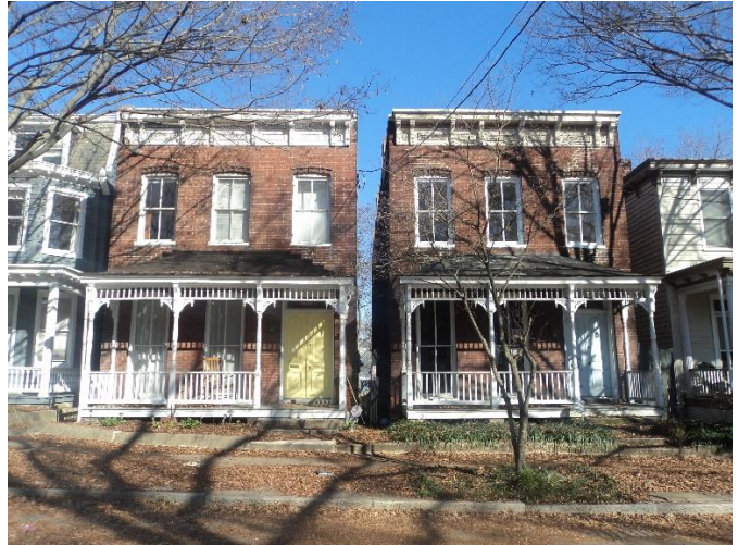
Figure 2. 3608 1/2 and 3610 East Broad Street.
