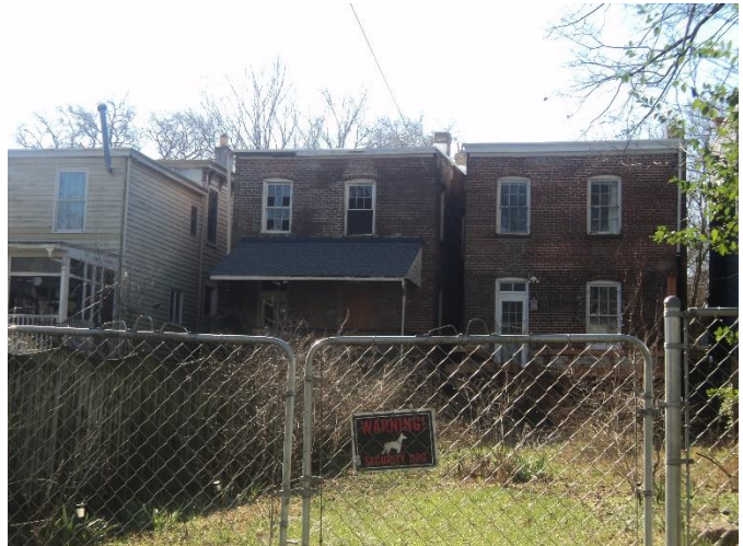
Figure 4. 3610 East Broad Street, rear elevation on left.
