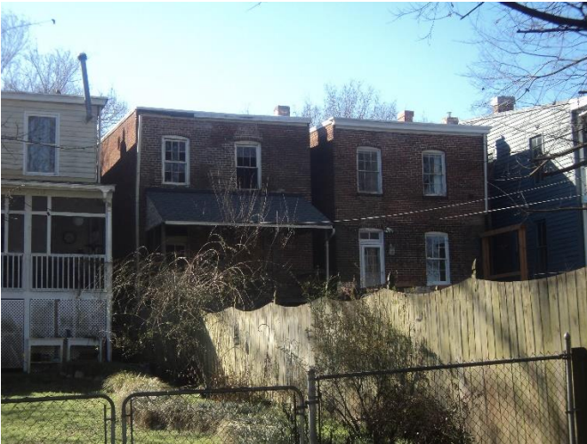
Figure 3. 3610 East Broad Street, rear elevation on left.
