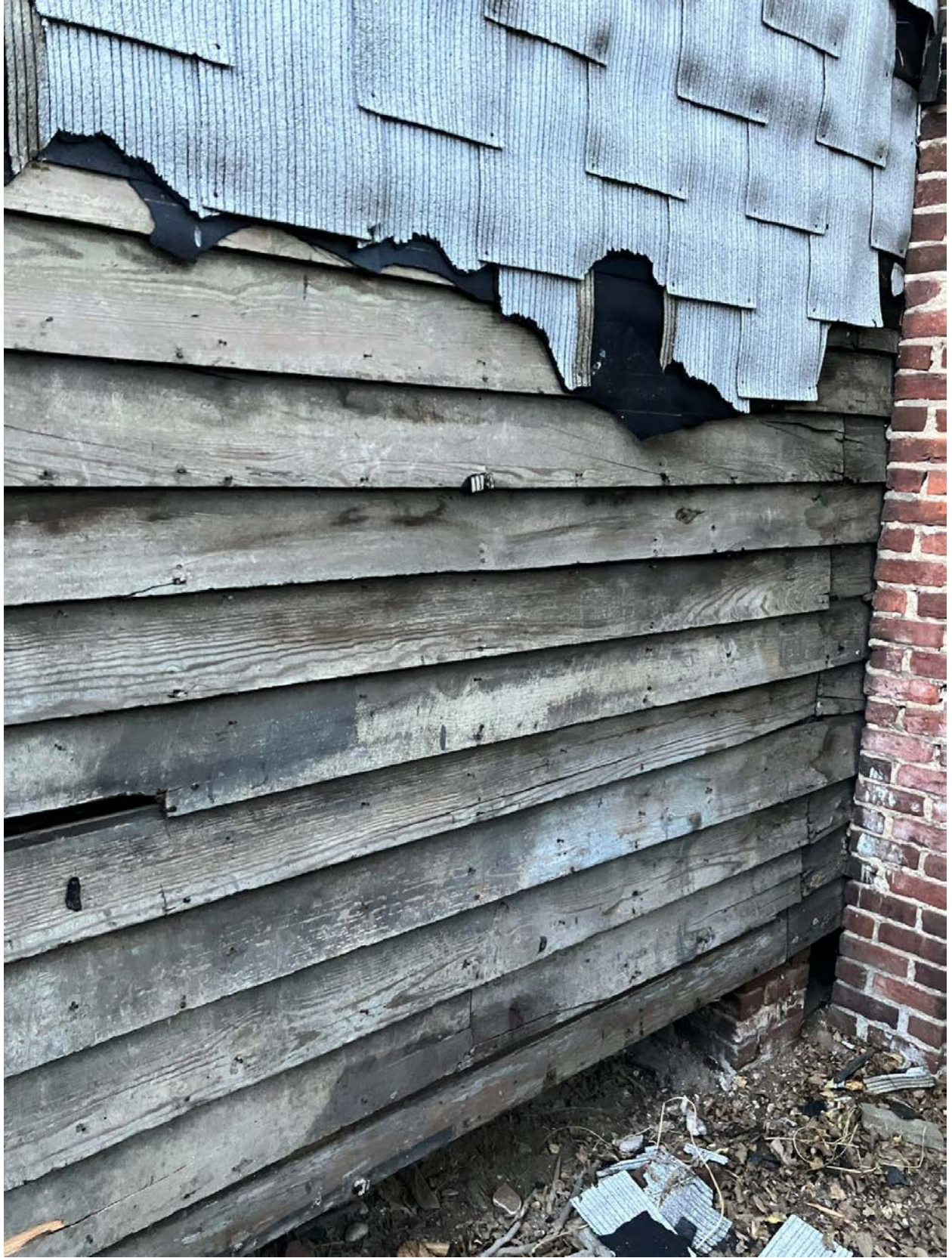
Image 13: Left side of house (side B) with original wood siding exposed.
