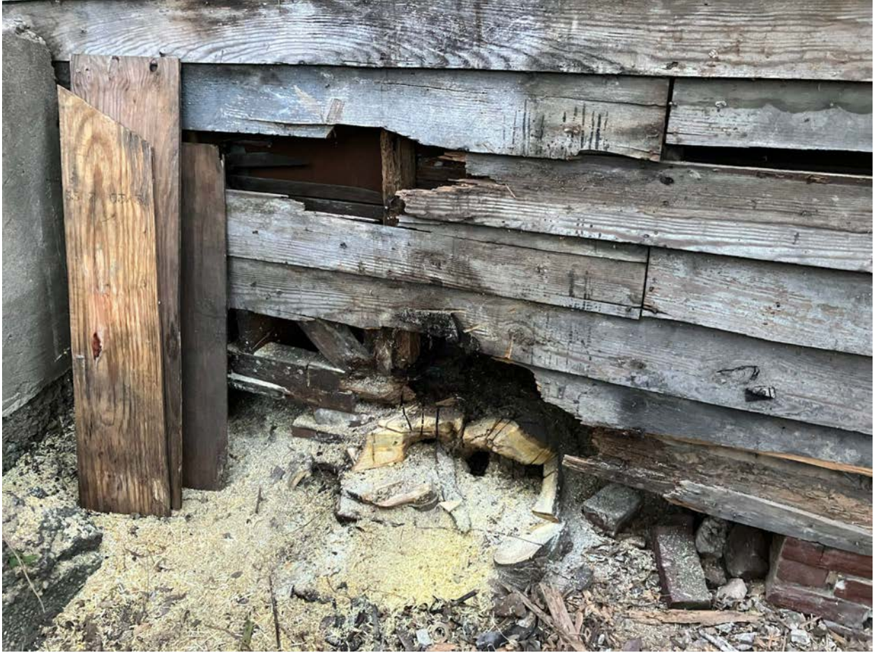
Image 12: Left side of house (side B) after stump removal; original wood siding has been exposed.
