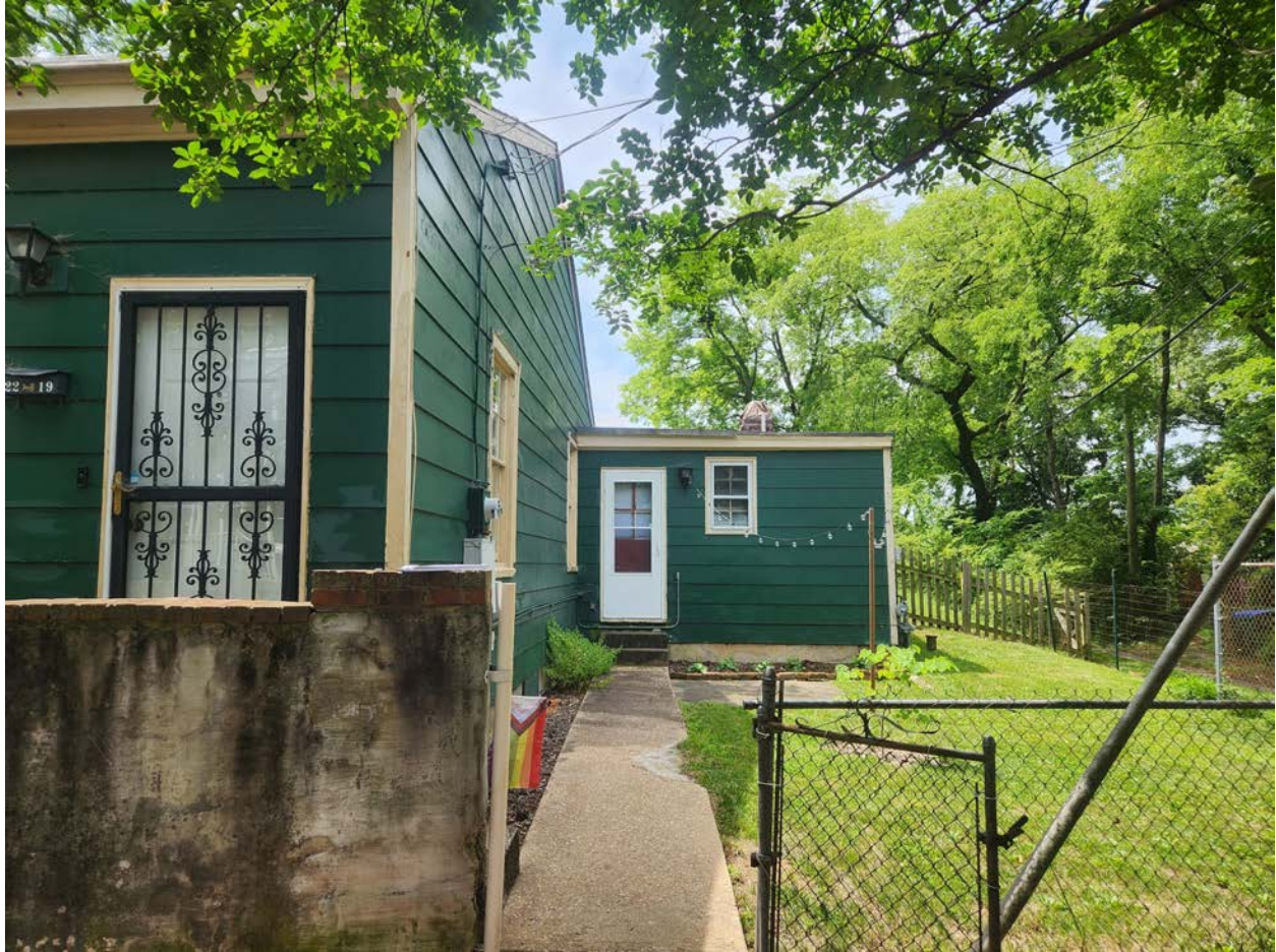
Image 3: Front elevation showing rear "extension" (side A)
