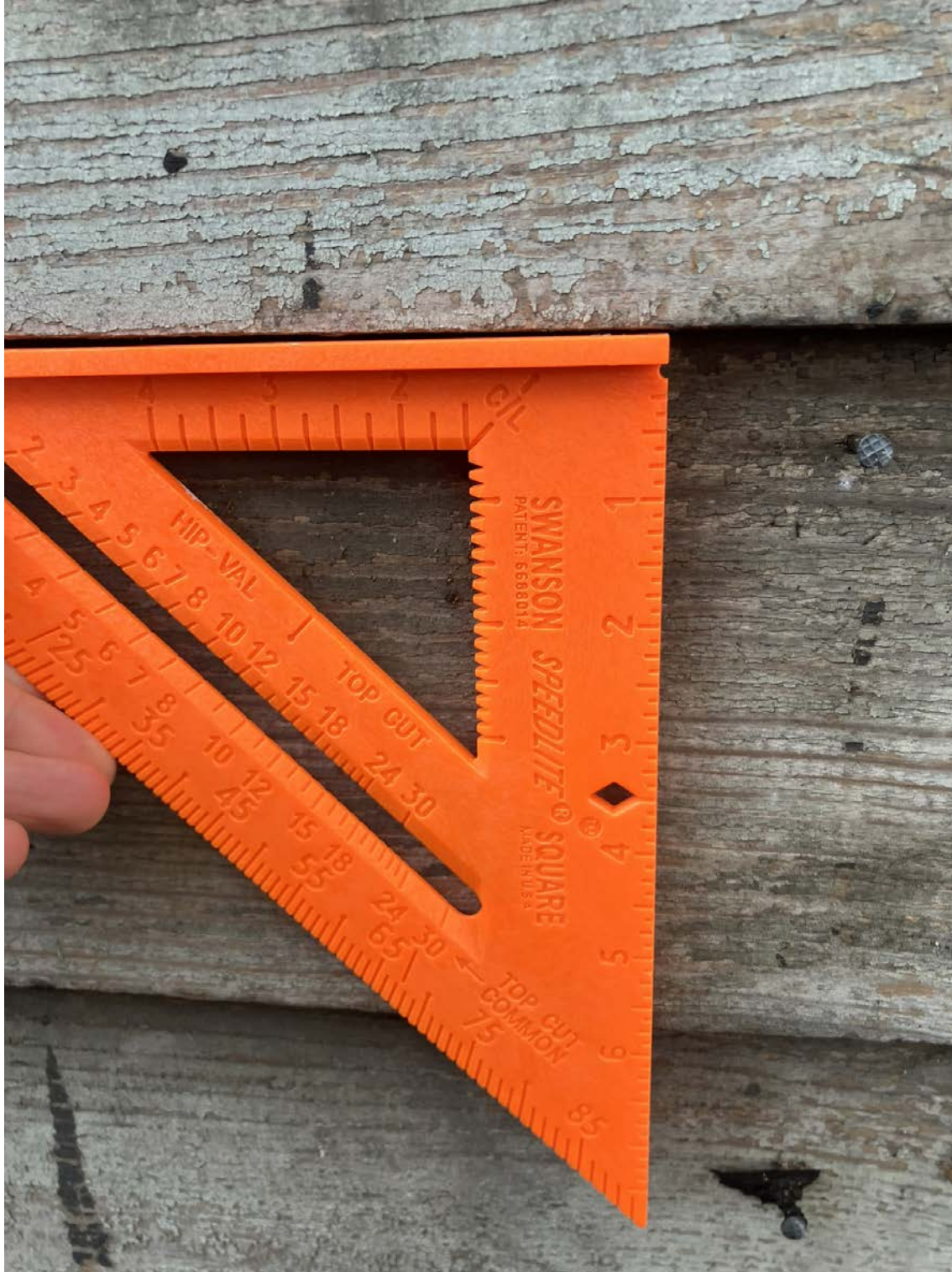
Images 15 & 16: Measurements of wood siding reveal shows that it's around 6" with some small variations.
