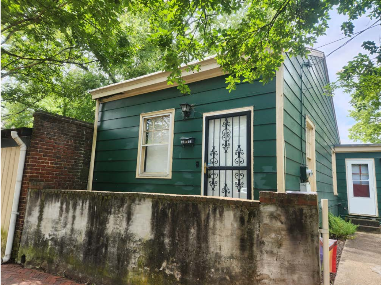
Image 1: Front elevation from M Street (side A)
