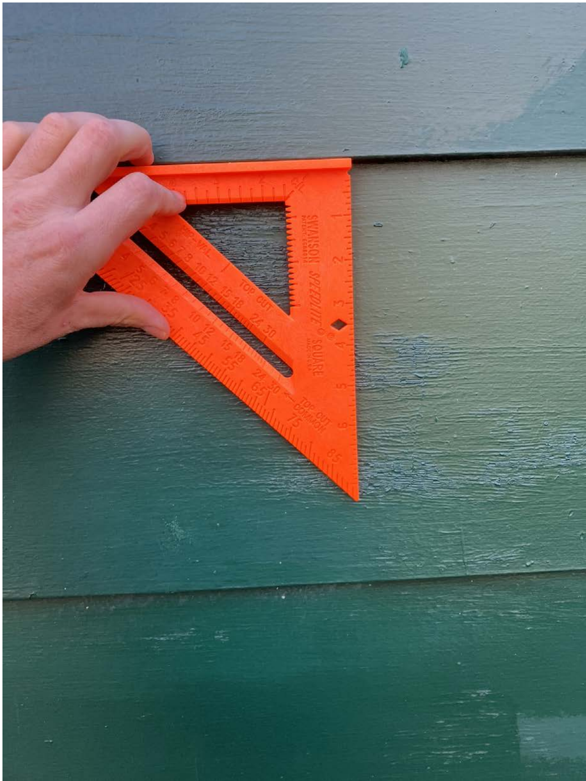
Image 17: Measurement of existing wood pressboard siding reveal.
