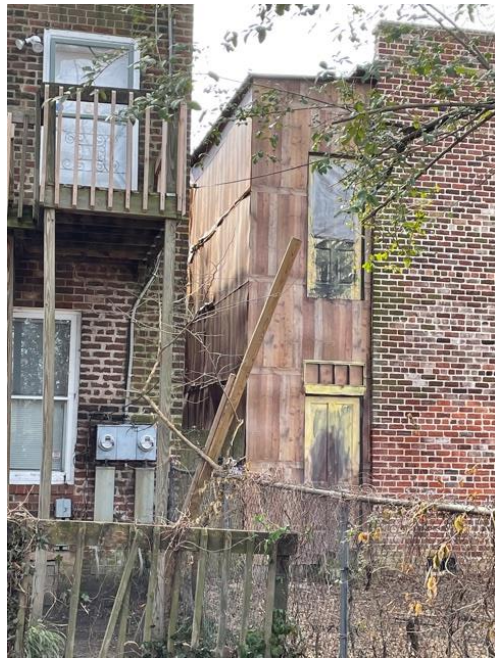
Figure 4. 316 W Leigh Street, ca. 2014 addition. .
