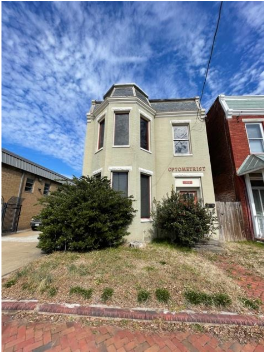
Figure 1. 316 W Leigh Street, facade.
