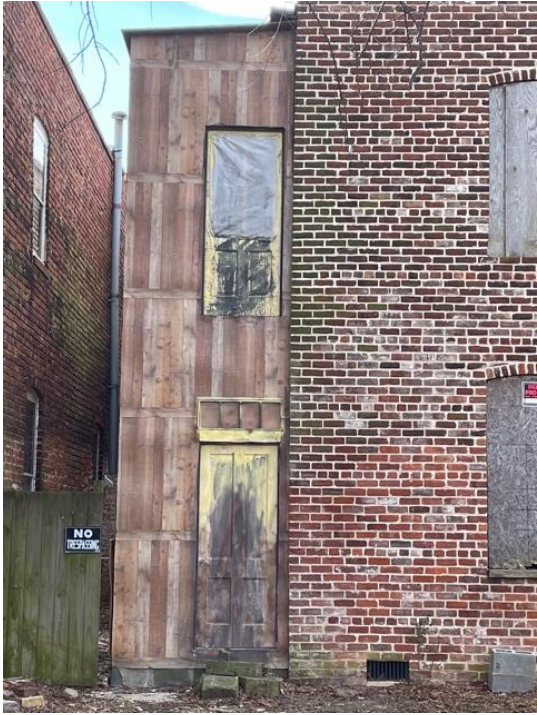
Figure 5. 316 W Leigh Street, addition existing openings. .
