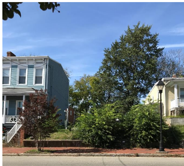
Figure 3. 910-912 North 25th Street
