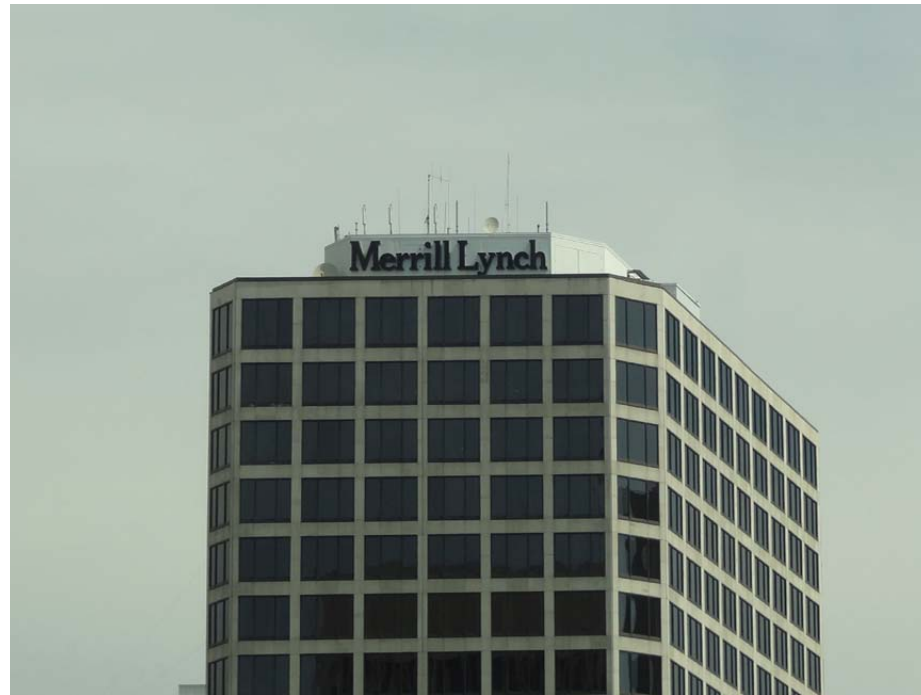
Existing Hi-Rise Building Letters - South Elevation
