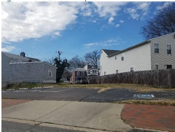
Figure 3. 803 Jessamine Street, view from across the parking lot at the rear.
