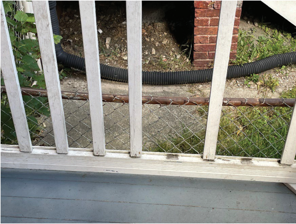
Photo #7: EXISTING CONDITION: Detail View #4 of deteriorating box column / base & porch fascia
