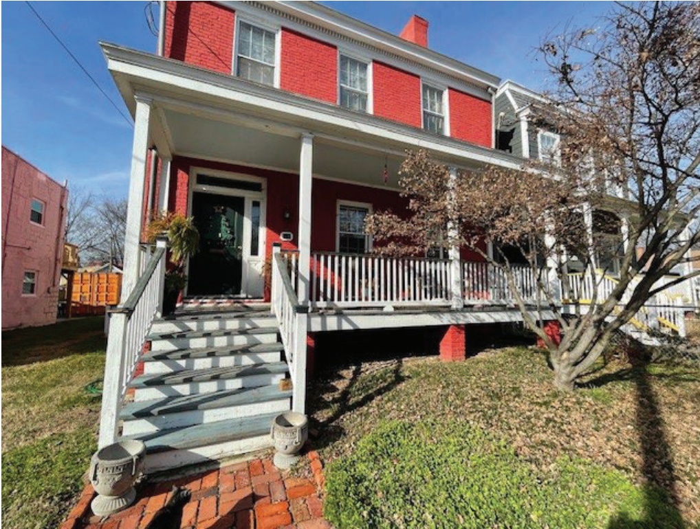
Photo #2: EXISTING CONDITION: Overall View #1 of front porch with existing Richmond Rail
