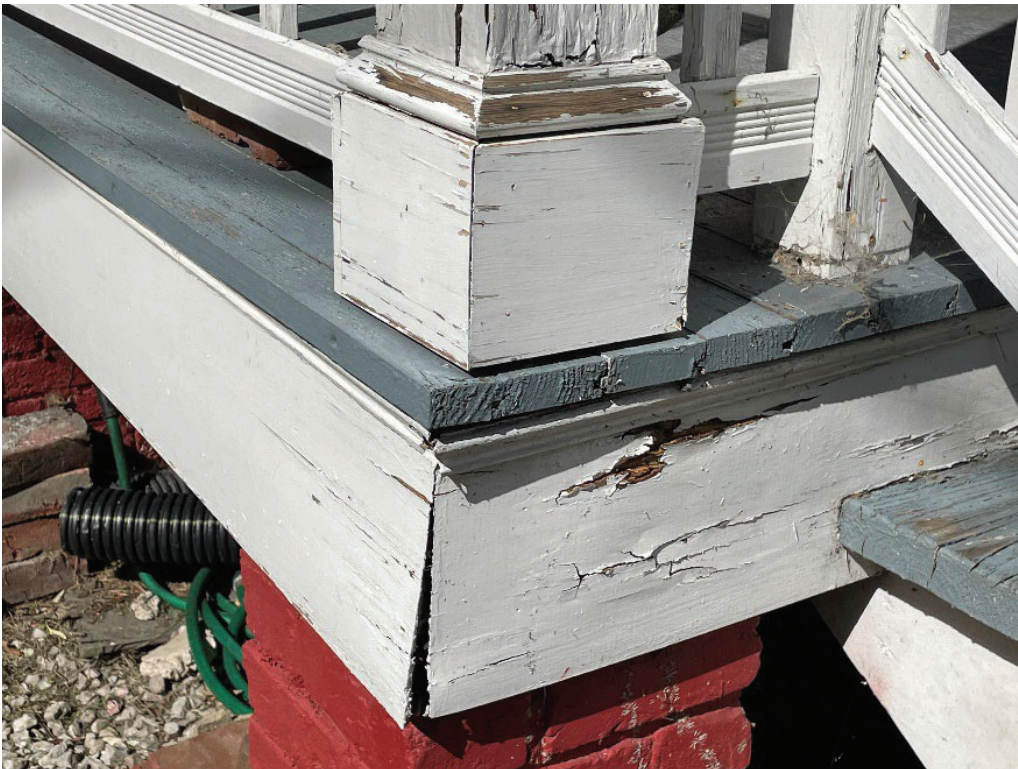
Photo #7: EXISTING CONDITION: Detail View #4 of deteriorating box column / base & porch fascia
