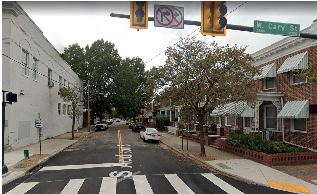
VIEW LOOKING SOUTH DOWN S. ADDISON STREET
