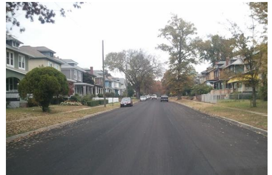
Completed Slurry Seal Application
