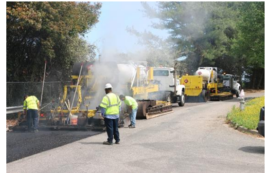
Heat Scarification Operation
