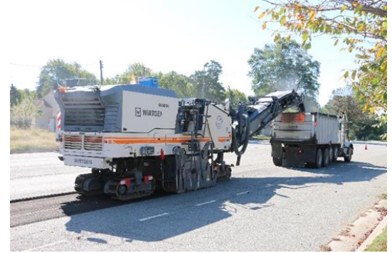
Milling and Overlay Operation
