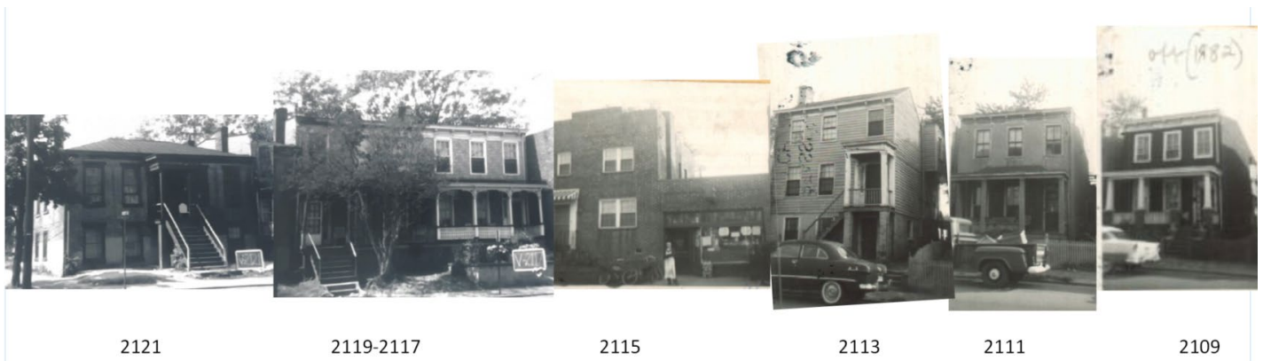
Figure 8. Subject block (2111-2119 Venable) in historic configuration, built-out. Photographs ~1955-1977. 2115 Venable picture below may not be the original building on that site.
