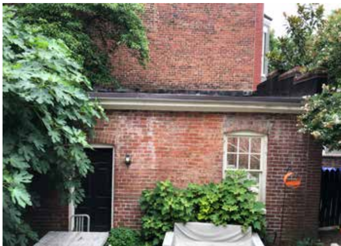
9 - WEST FACADE OF ACCESSORY STRUCTURE
