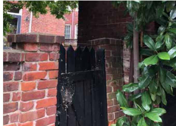
10 - INTERIOR BRICK WALL / GATE
