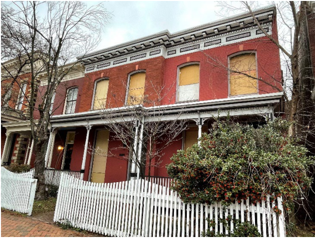
Figure 1. Façade of 2616 East Grace Street
