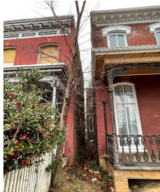
Figure 4. View of the small gap between 2616 and 2620 East Grace Street. The rear projection of 2620 East Grace Street can be seen in the back of the image, conveying that the proposed addition will not be visible from East Grace Street.
