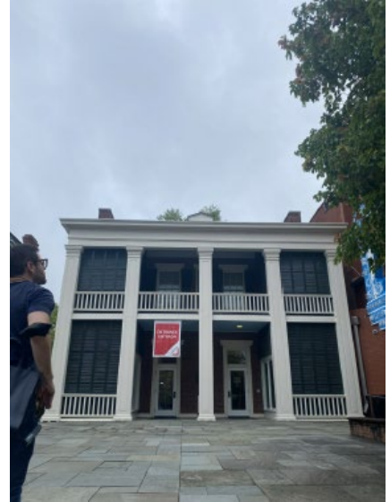
Figure 2. View of rear of Bransford Cecil House.
