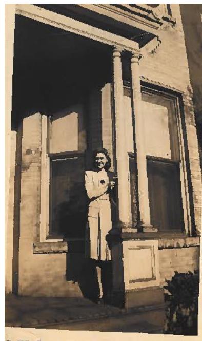
Figure 8. 2010 West Grace Street, column detail, undated photographs provided by the applicant.
