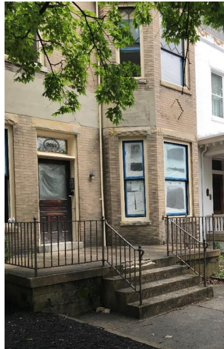
Figure 4. 2010 West Grace Street, side view of facade
