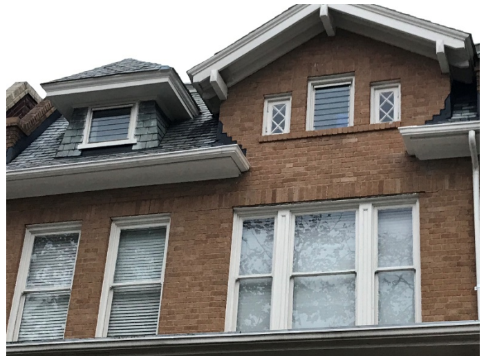
Figure 2. Windows, existing condition.
