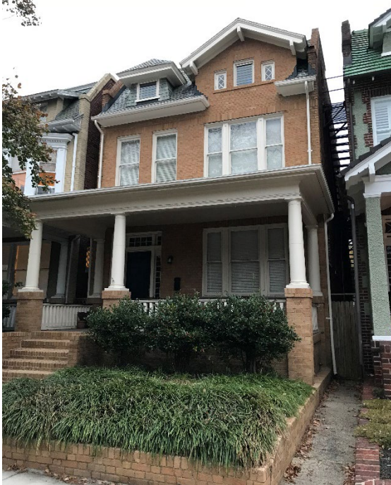
Figure 1. 109 North Arthur Ashe Boulevard, façade.
