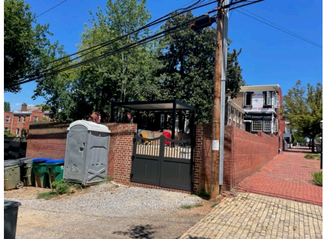
Figure 2. View of pergola and rear yard looking north from rear alley. Newly installed gates partially obscure the rear yard.
