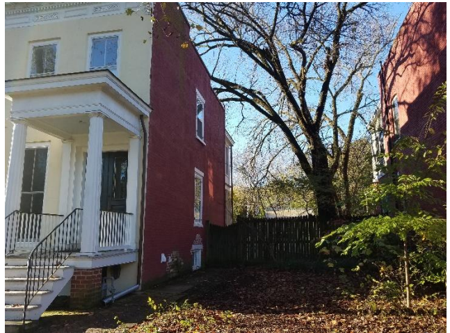
Figure 4. View towards project location from East Broad Street.
