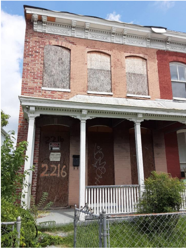
Figure 1. 2216 Venable Street, façade
