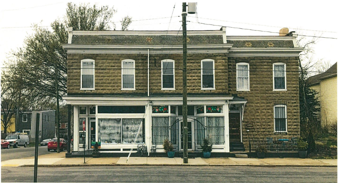
600 north 29th street | corner commercial space due west of proposed home
