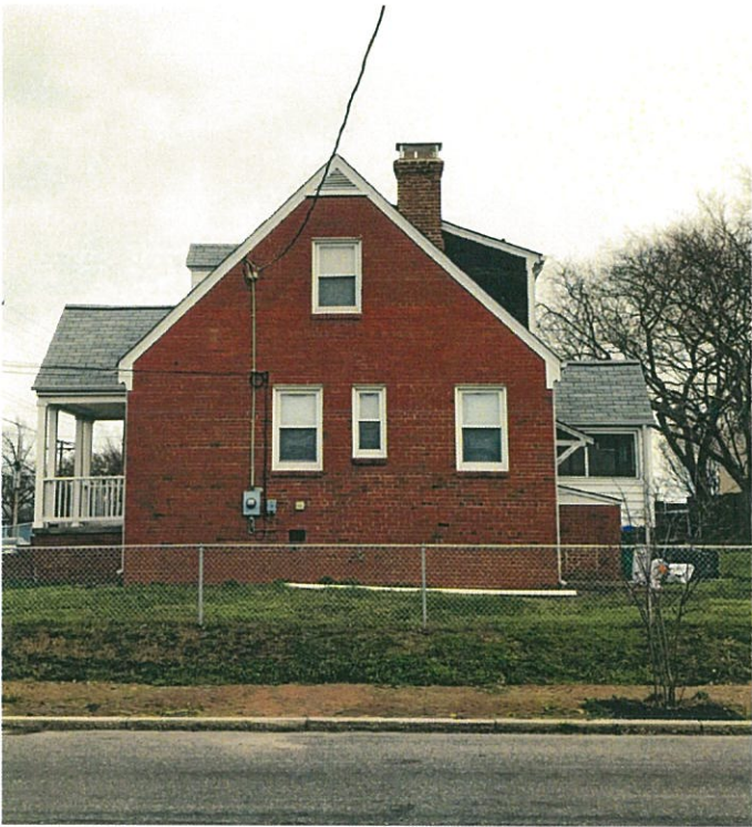
2901 m street | gable facing north 29th street
