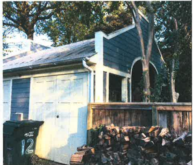
Carriage house with end wood parapets, sloped with chimney shape at peak; 14 N. 30 th Street
