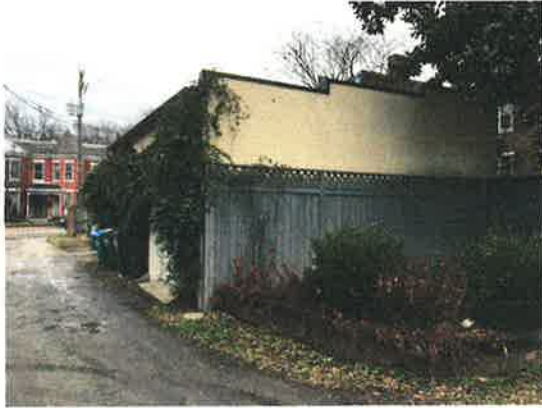
Garage with stucco finish, cream color; 318 N. 24 th Street
