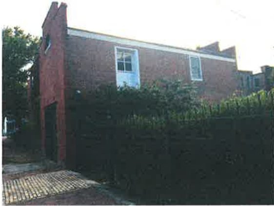
Carriage house with end masonry parapets, stepped, with gable roof behind; 2618 East Broad Street
