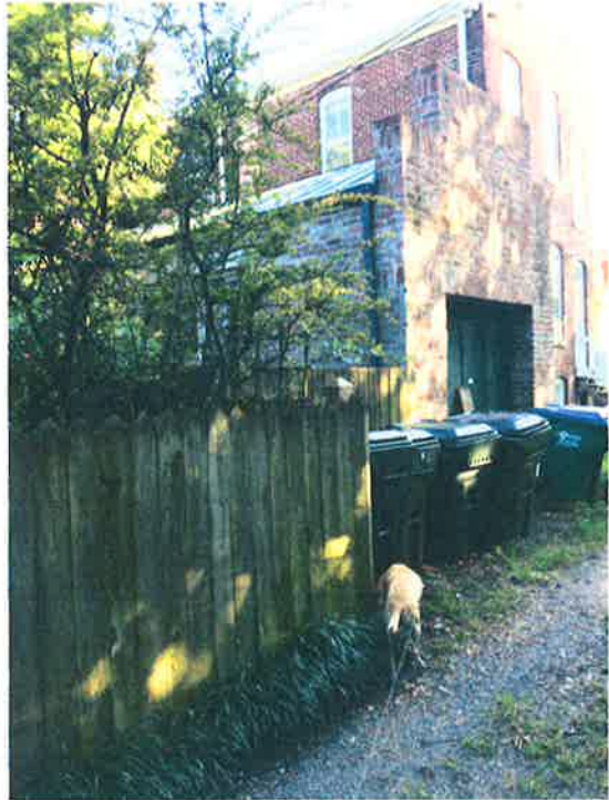
Carriage house with end masonry parapets, stepped, with gable roof behind; 1 North 29 th Street
