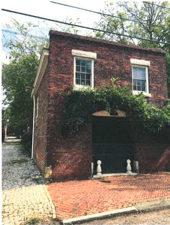
Carriage house with end masonry parapets; 2200 East Grace Street
