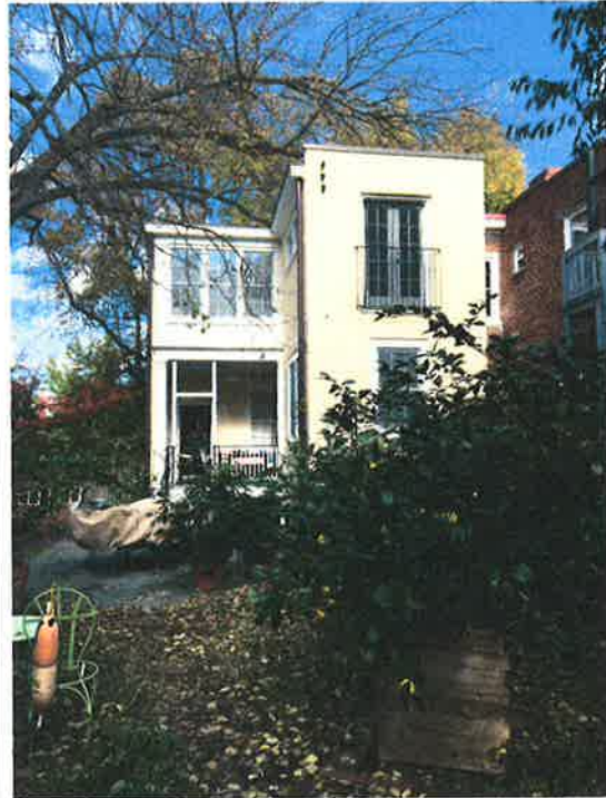
Stucco finish on main home at 2711 East Broad Street – rear, to cover cinderblock (approved by CAR in 2009)
