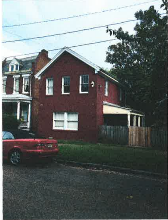
Accessory residence with masonry gable end and gable roof with overhang; 2800 East Grace Street
