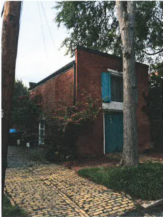
Carriage house with end masonry parapet; 2717 East Grace Street
