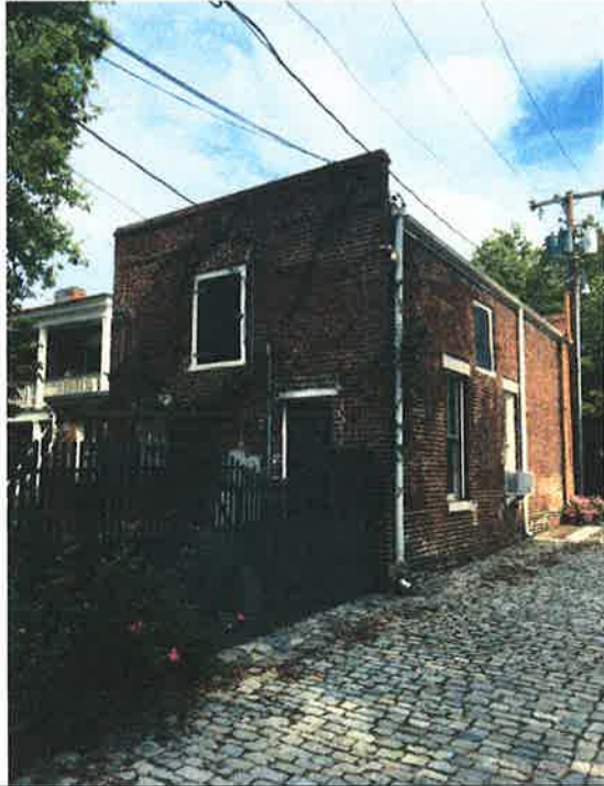
Example of asymmetrical window and door arrangement; 210 N. 23 rd Street
