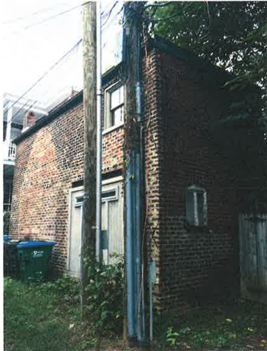
Example of square windows on side, and asymmetrical window configuration on rear; 2707 E Broad Street
