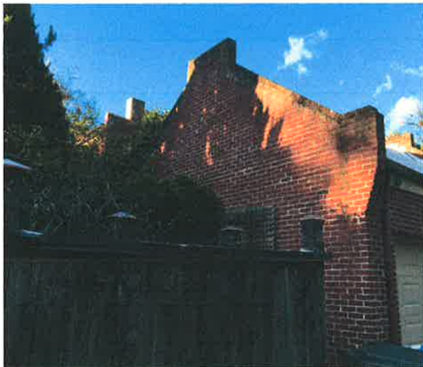
Garage with end masonry parapet, sloped with chimney shape at peak, gable roof behind, 2708 E. Grace Street
