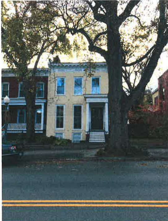
Stucco finish on main home at 2711 East Broad Street – front
