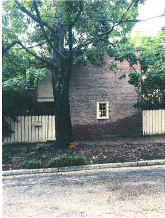
Example of small vertical window reflecting proportions of our second-floor windows on rear, east, west facades; 101 N. 28 th Street
