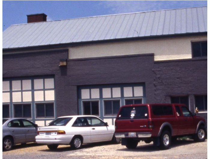
Figure 2. Rear garage at 211 North 18 th Street. Second-story addition constructed without skylights.
