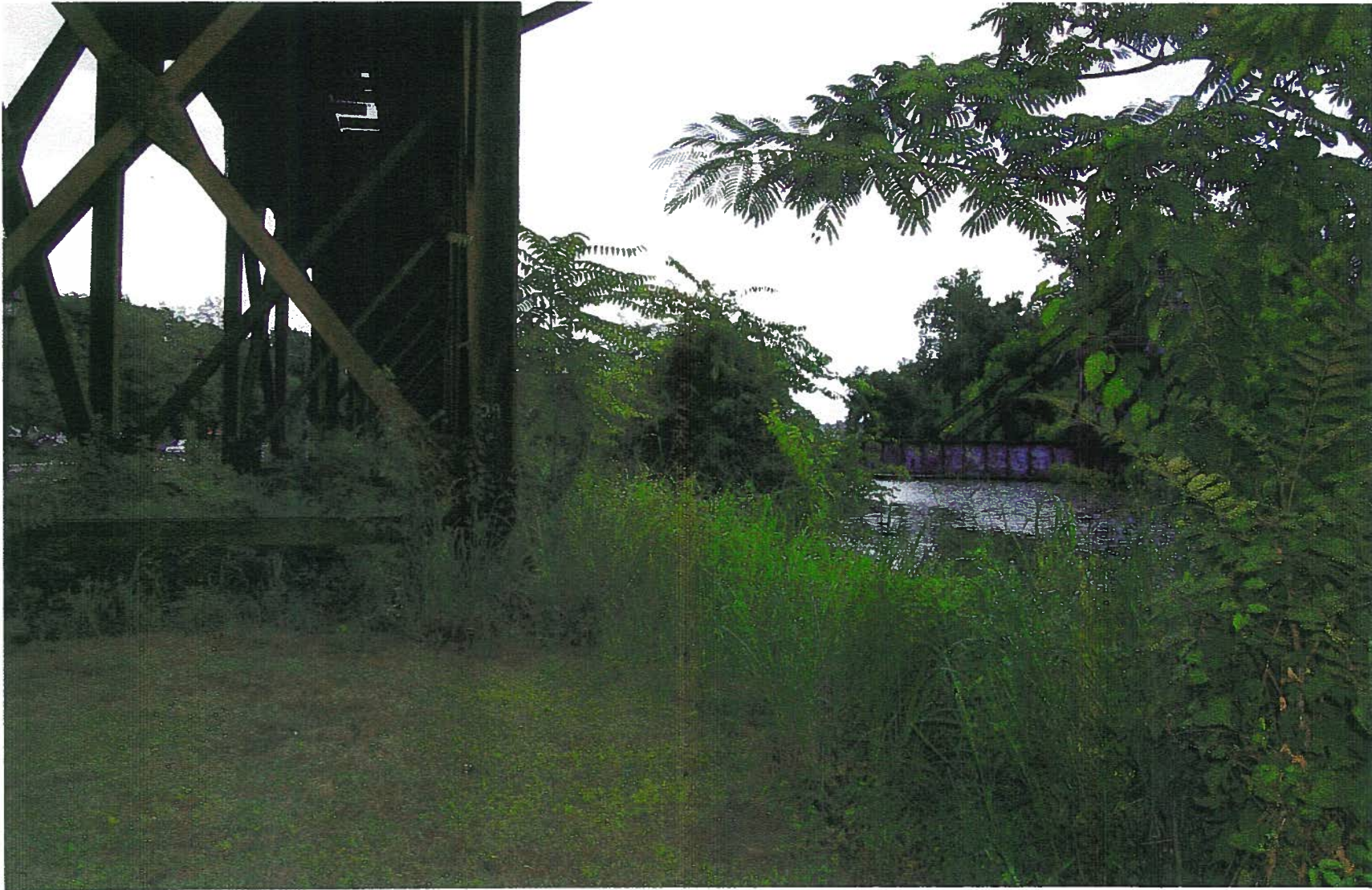
LOW LINE DOCK WALK (E) - EXISTING CONDITION
