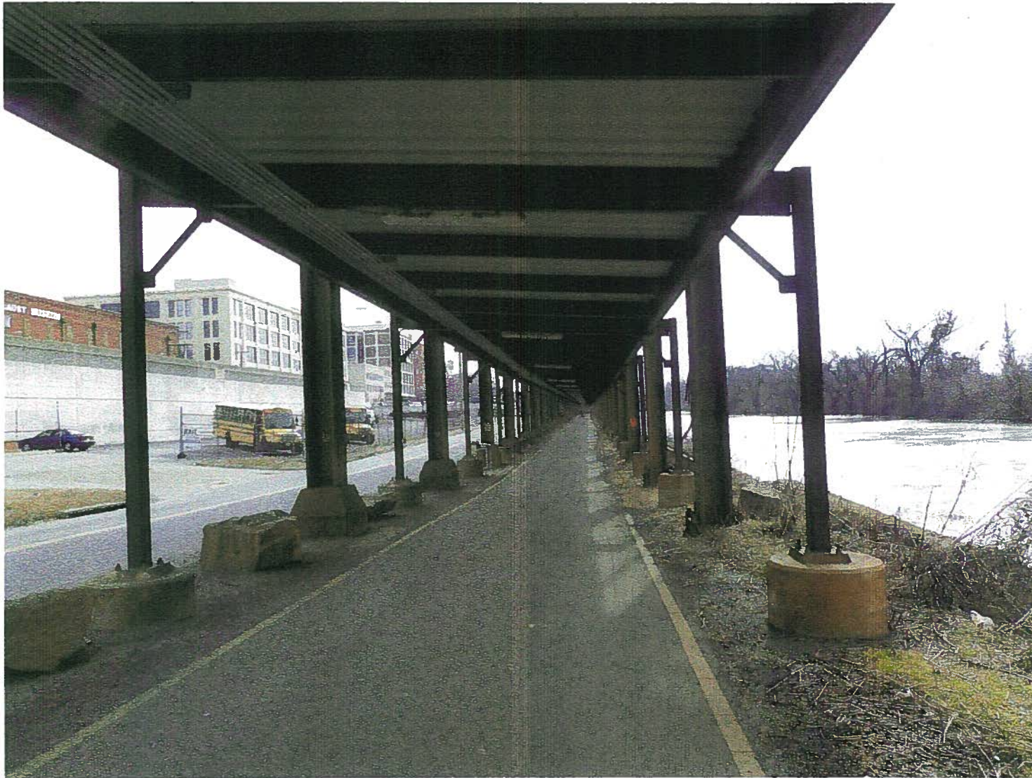
CAPITAL TRAIL CROSSING (C) - EXISTING CONDITION
