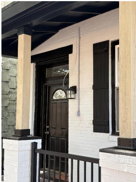
Figure 3. New square posts installed on the front porch, secured with brackets and bolts.
