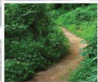
Compacted Earth Trail 3'-0" wide
