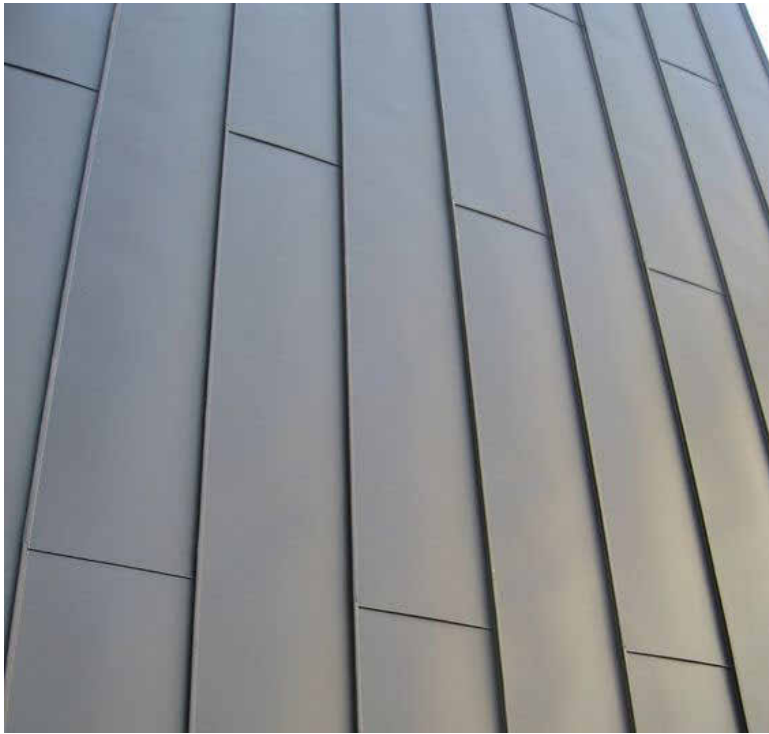
ZINC STANDING SEAM ROOF
