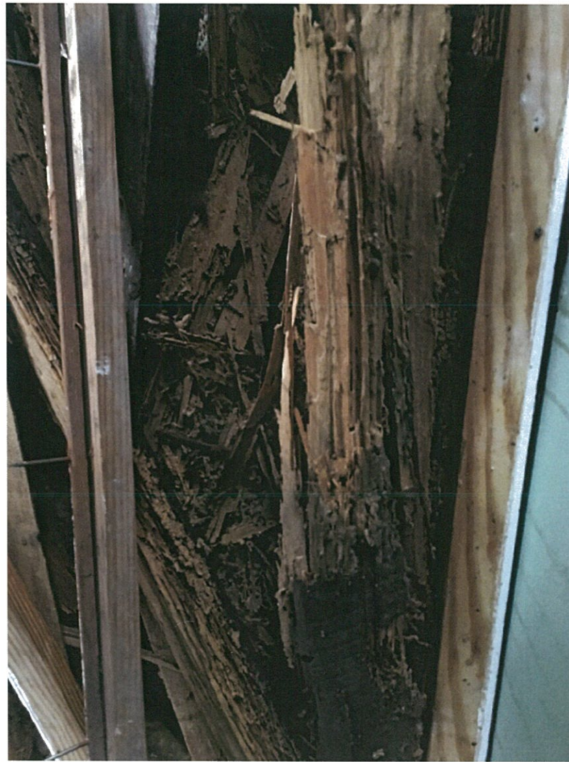
Existing Rear Section, Photograph 7
