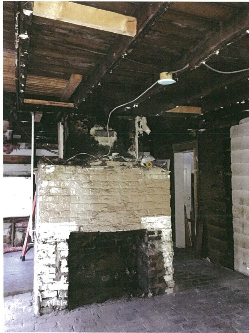
Existing Rear Section, Photographs 1 & 3 - 1st level north section
