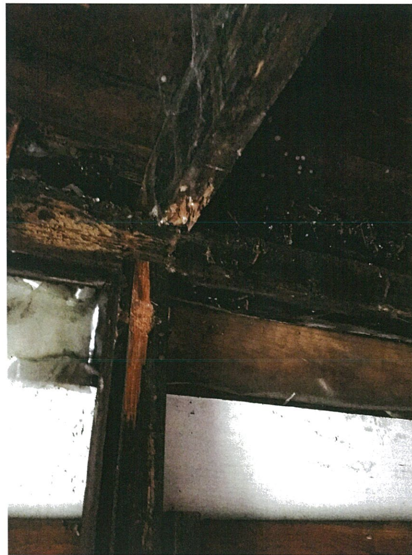
Existing Rear Section, Photograph 8
