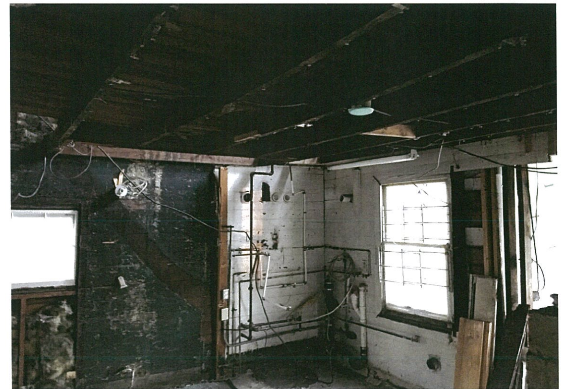
Conditions within the rear, shed roof, section:
