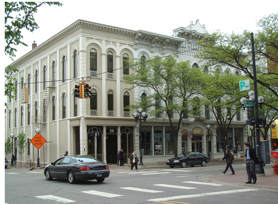
Goodyear Building, Ann Arbor's First PACE project
