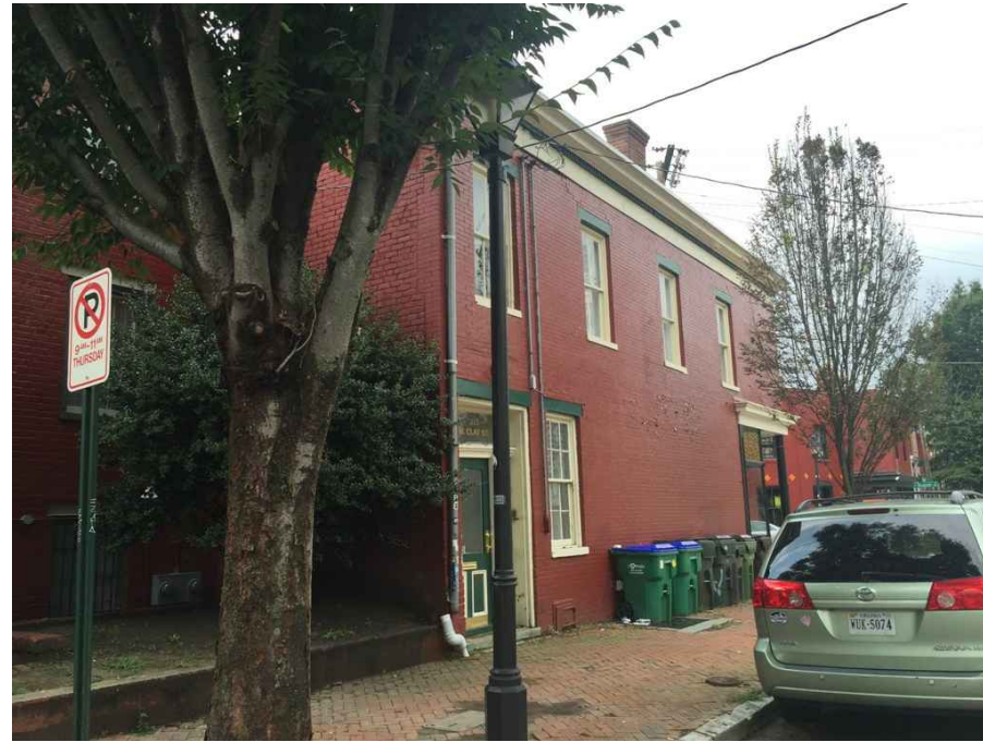
w clay st view from east
