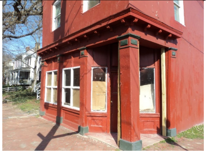
Figure 2. Corner detail, April 2018.
