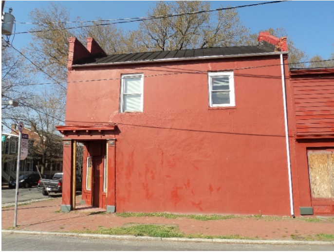
Figure 1. South wall, April 2018.
