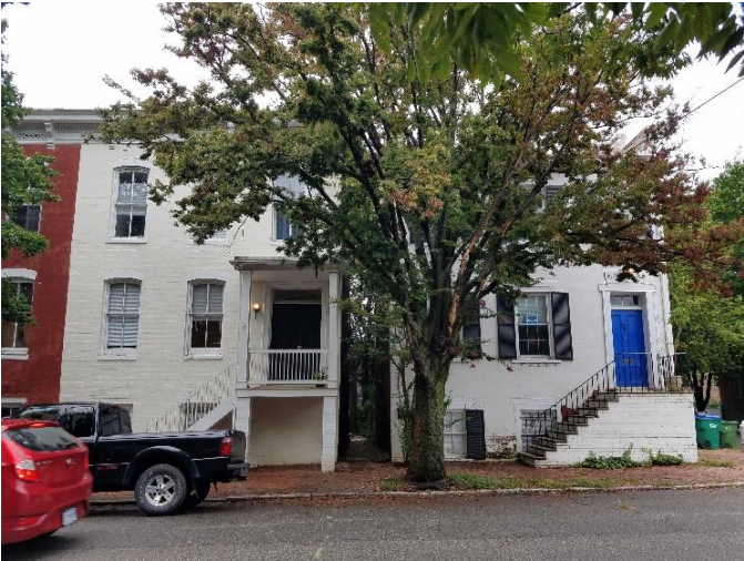
Figure 7. 2322 and 2324 E. Marshall Street.
