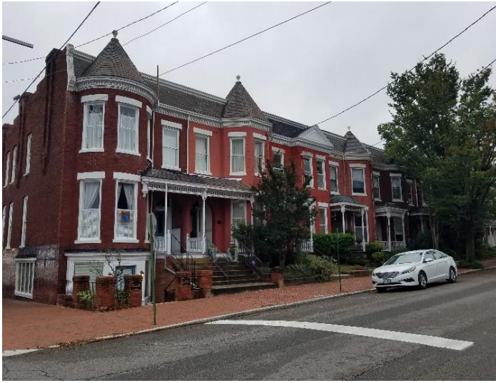
Figure 9. Adams Row, 2300-2316 E. Marshall Street.
