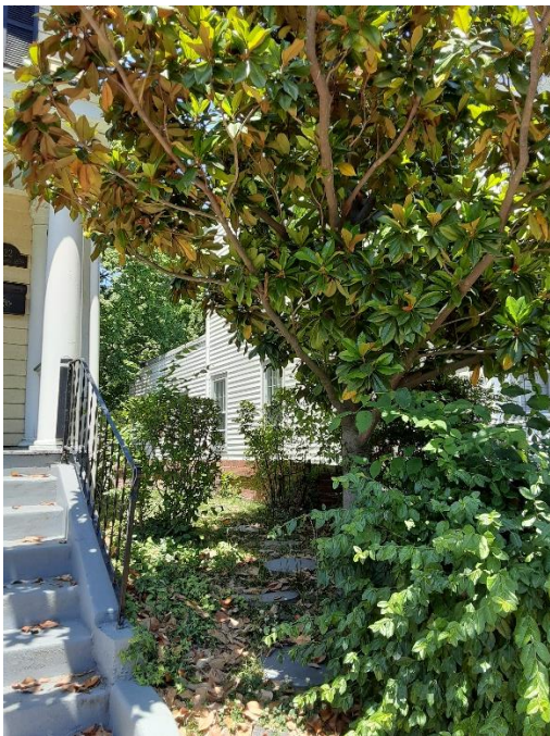
Figure 3. View towards existing rear section and location of proposed addition.
