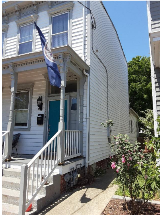
Figure 2. View towards existing rear section and location of the proposed addition.
