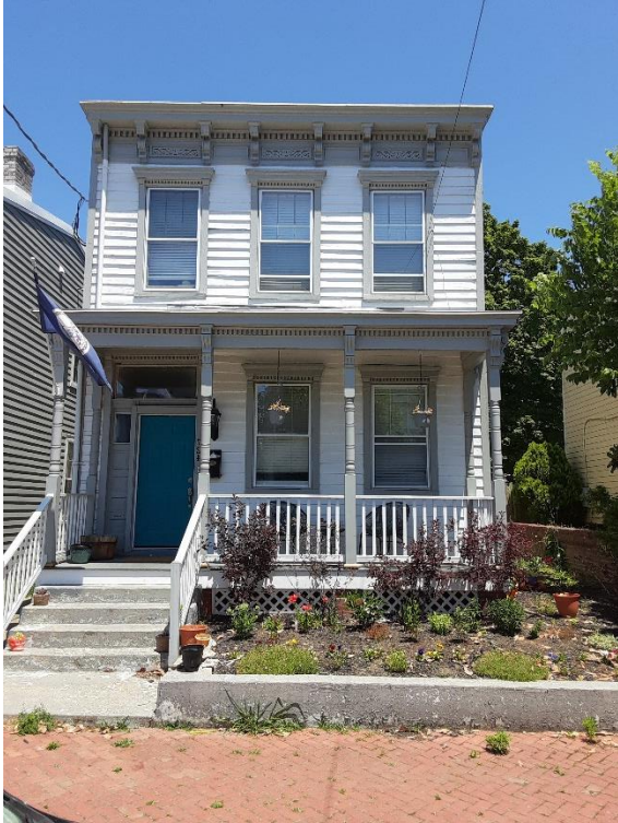
Figure 1. 724 N. 27th St, facade.
