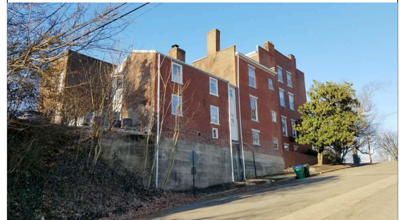
N 29TH ST. HOUSE ACROSS STREET
