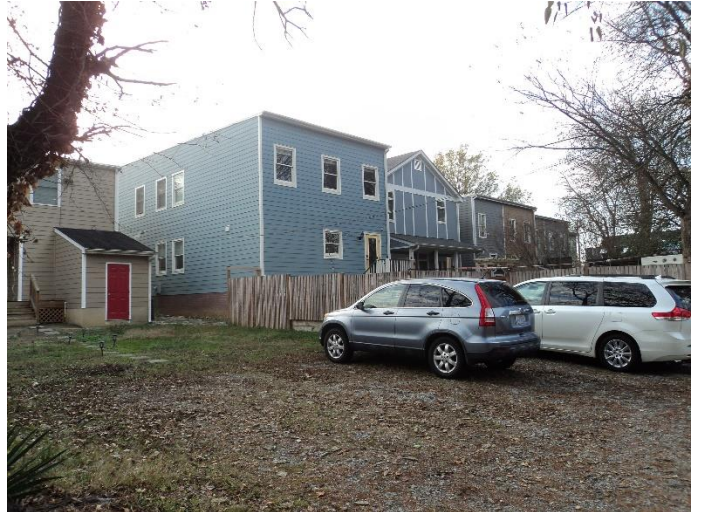
Figure 2. 514 North 28th Street, north and west elevations.
