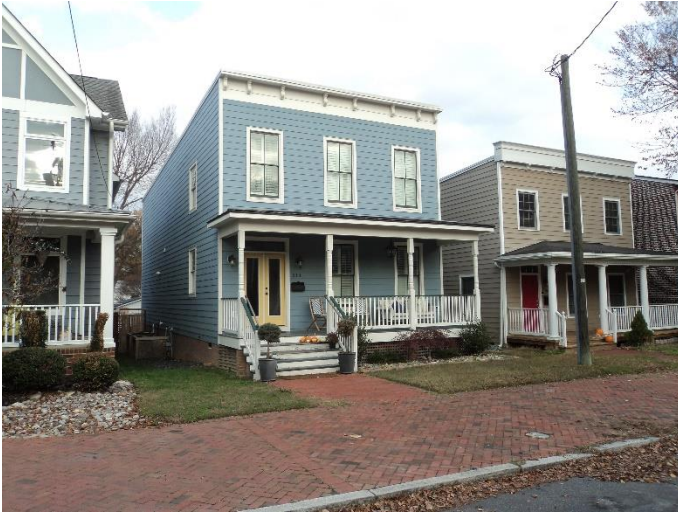
Figure 1. 514 North 28th Street, south and east elevations.
