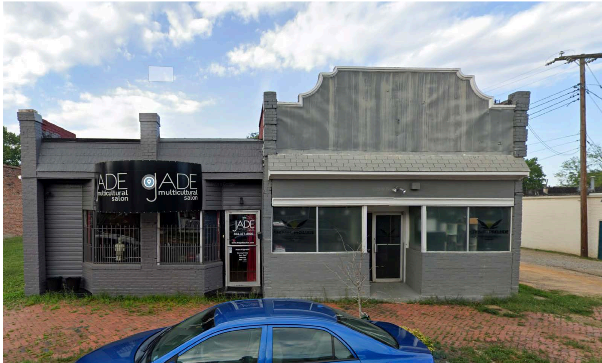
3304 and 3306 E Marshall St commercial fronts prior to demolition
