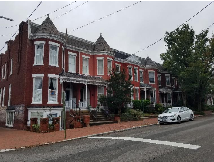
Figure 3. Adams Row, 2300-2316 E. Marshall Street.
