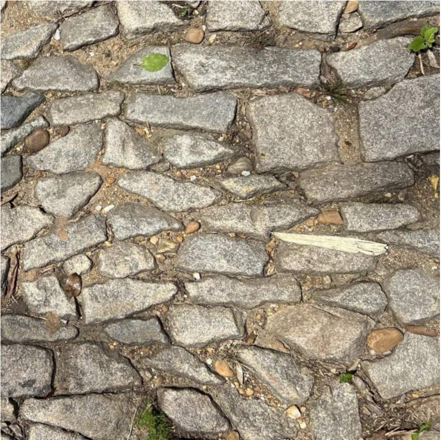
Existing cobblestone from pathway adjacent to the side facade new cobblestone area to be build using existing extra cobbles on site from previous drive modification
