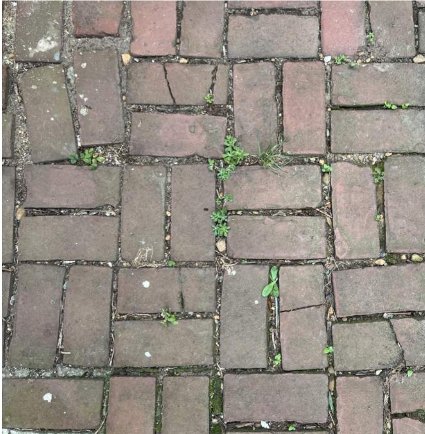
Existing brick from back facade exterior floor infill brick at patio to be built using extra bricks on site from previous patio modification
