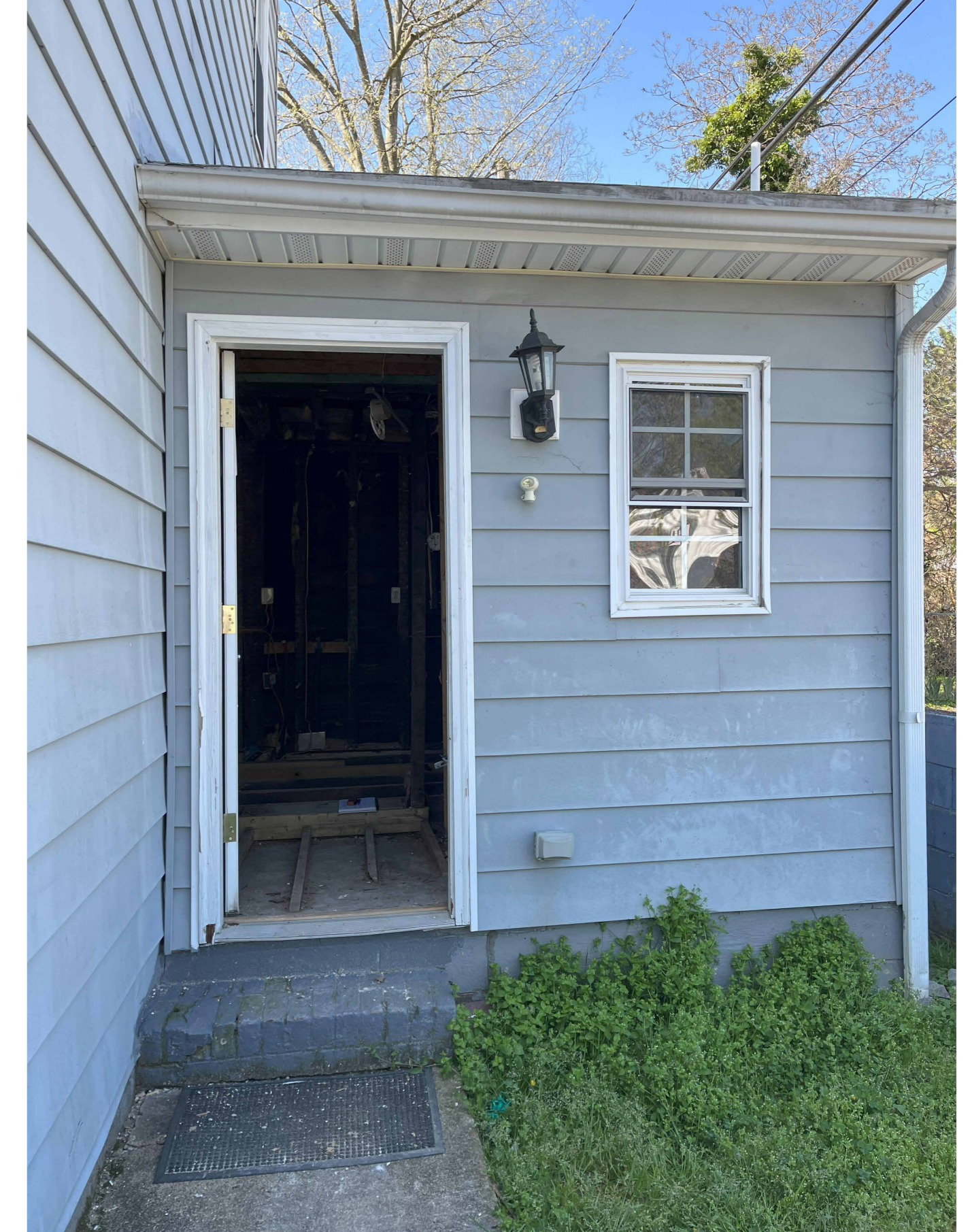
EXISTING ONE STORY ADDITION
