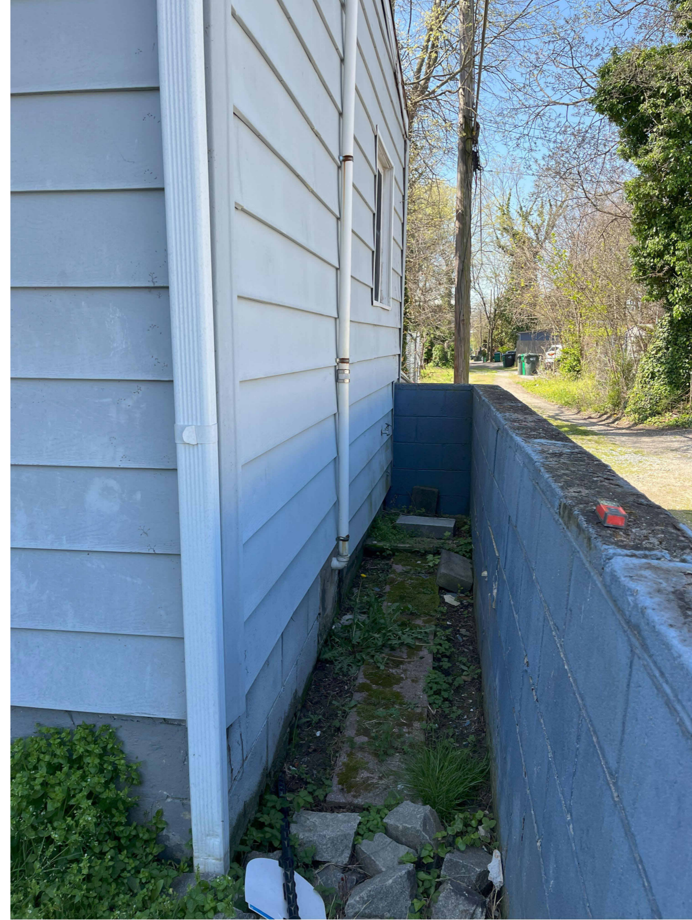
EXISTING SITE WALL AT ALLEY
