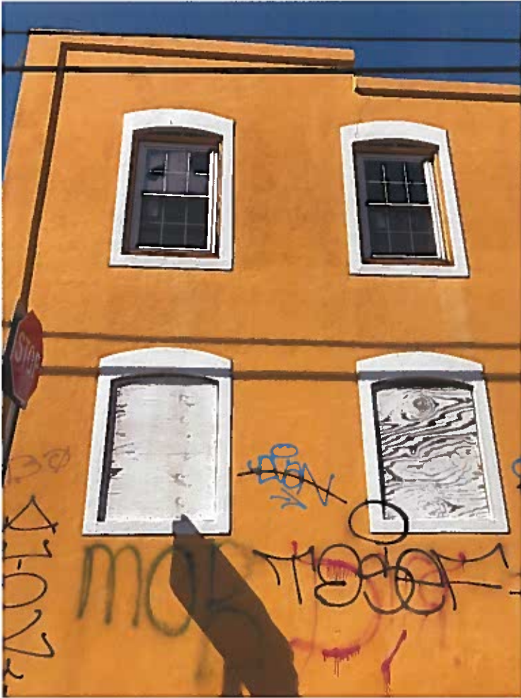
815 N 22 nd Street - historic window openings
