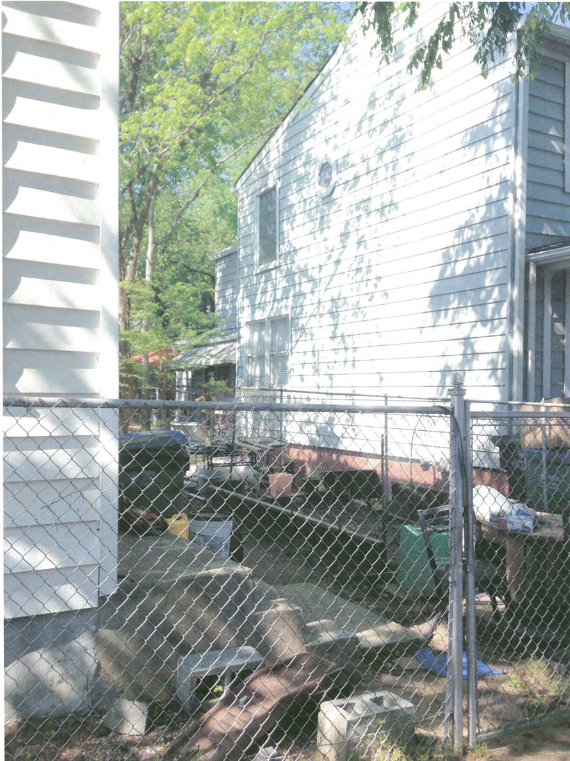
View of the proposed work site from East Clay Street A portion of the existing/proposed addition will be visible from the public right-of-way.
