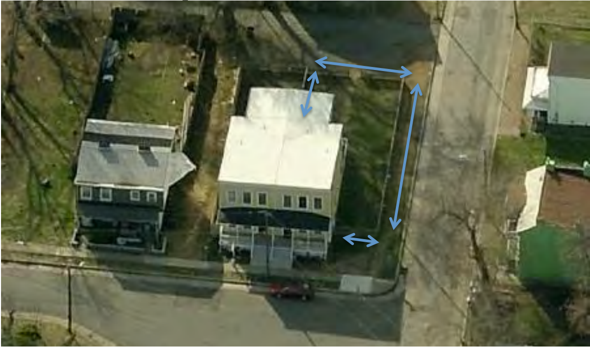
978 Pink Street is the attached single-family house on the corner. There are approximately 175' of 3.5' wooden fence as shown via arrows above.
