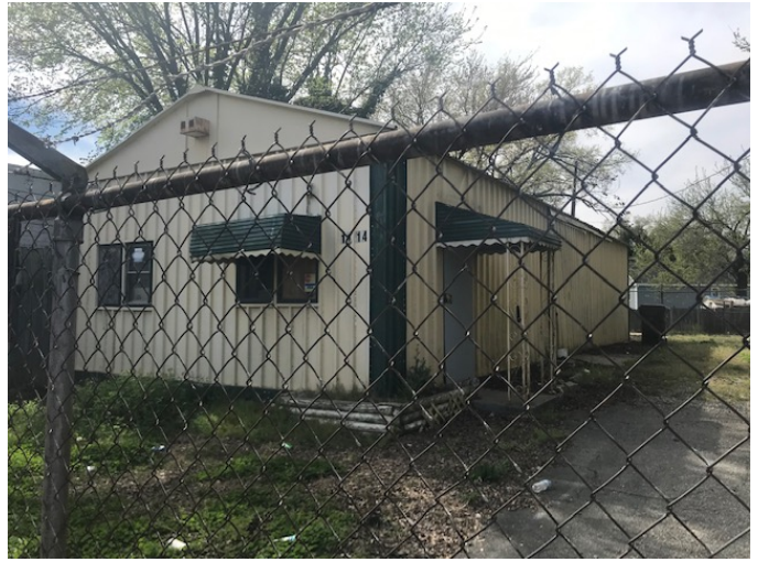
Figure 2. 1114 North 25th Street, existing building.
