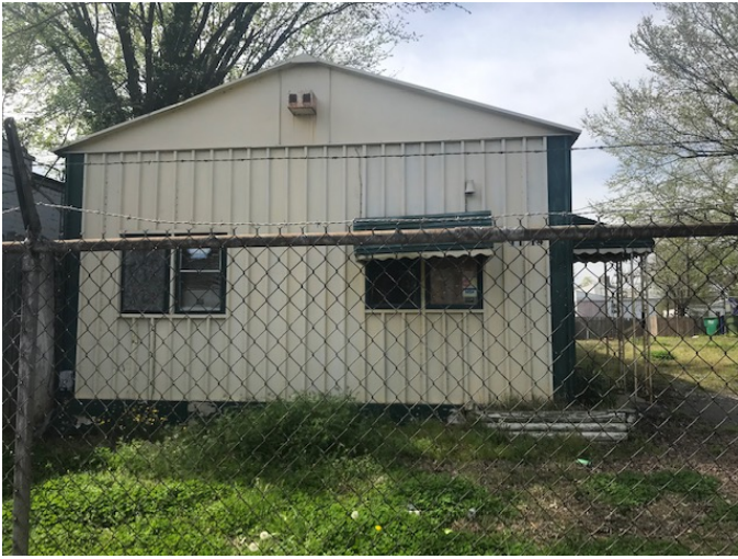
Figure 1. 1114 North 25th Street, existing building.
