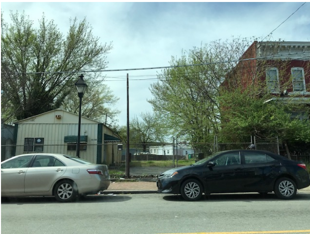
Figure 3. 1114 North 25th Street.
